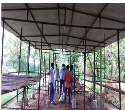
Installation of Onion storage structure at Ganrei village
