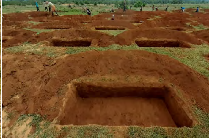
Staggered Trench at Haldi GP
