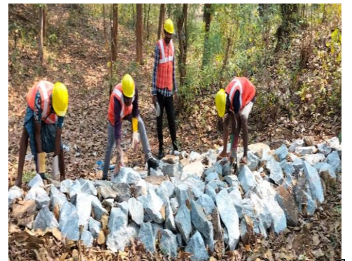
Construction of LBS
