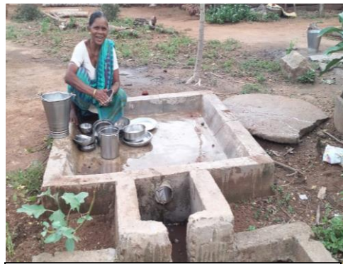
Construction of soak pit under grey water management
